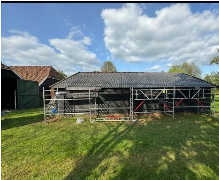
Installing New Roof Tiles.
