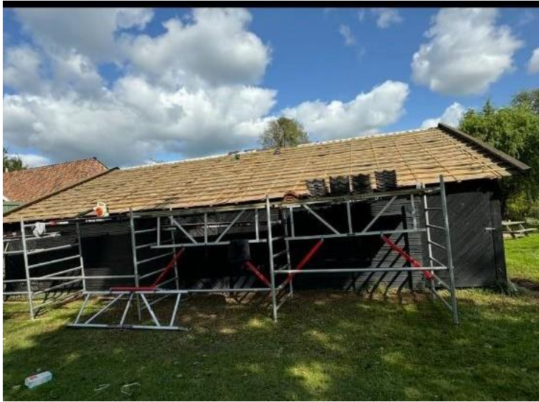
Laying new roof tiles ready.
